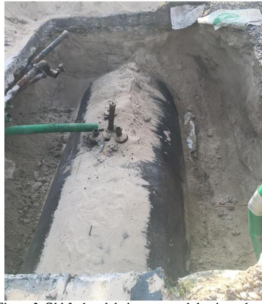
**Figure 3:** Old fuel tank being removed that is enclosed in sand.
